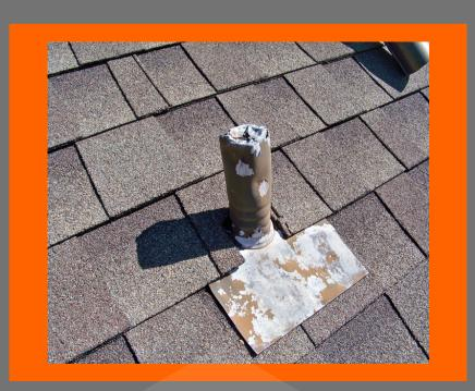
Other companies use lead pipe jacks, which lead to deterioration, leaks, and provide an entry point for small animals that may cause infestations...
