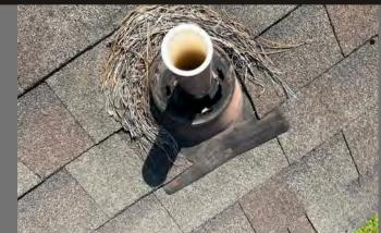
Other companies use lead and rubber pipe jacks, which lead to deterioration, leaks, and provide an entry point for small animals that may cause infestations...
